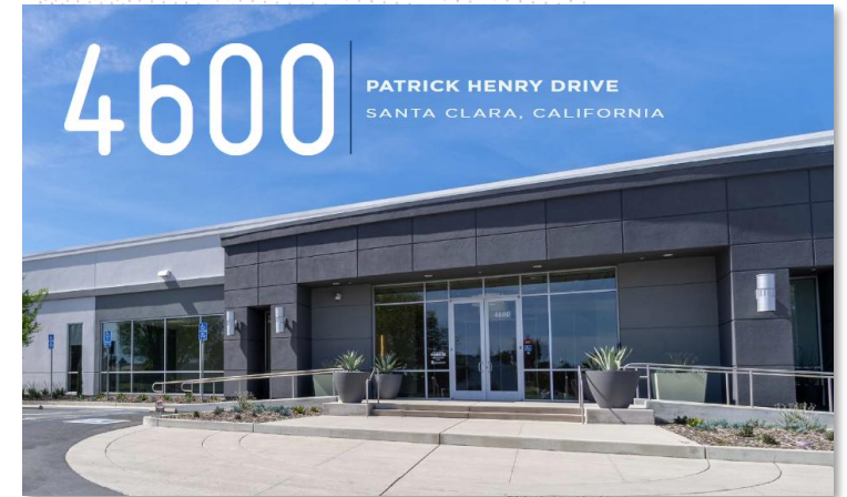
State-of-the-art facility in Santa Clara, California
