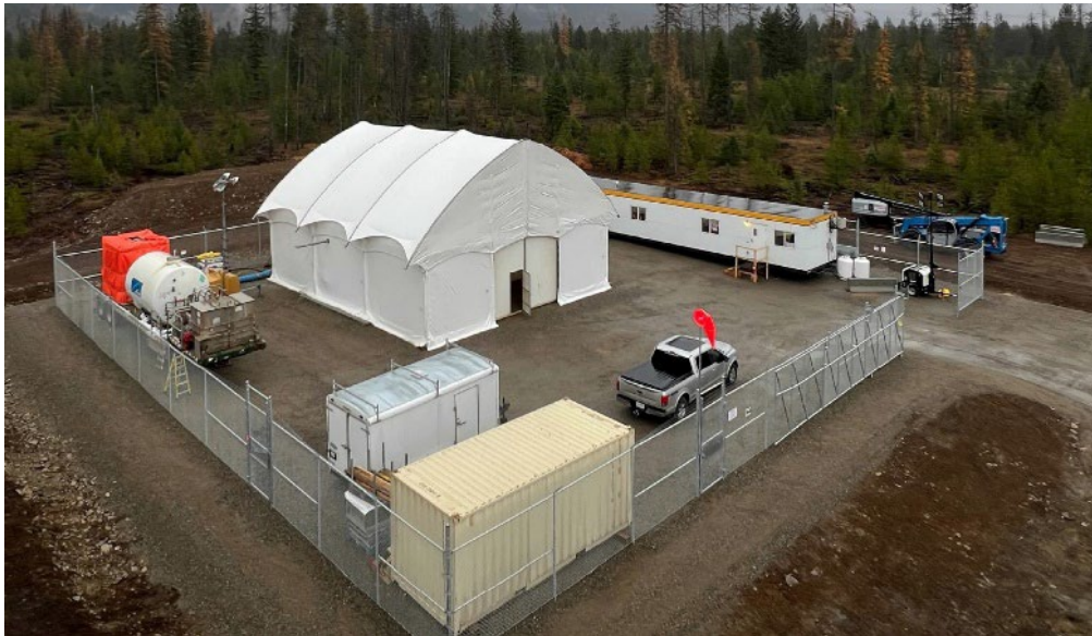
FortisBC test rig site in BC, Canada
