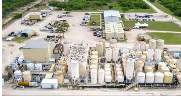
Alta Mesa Central Processing Plant, Texas, USA
