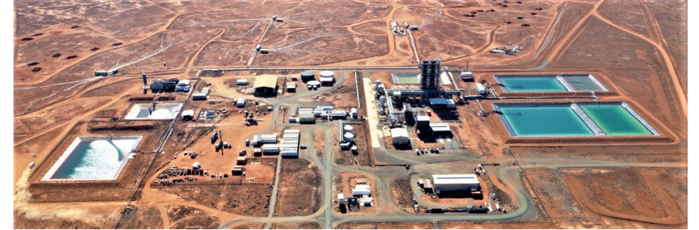
Honeymoon Processing Plant and Wellfields, South Australia
