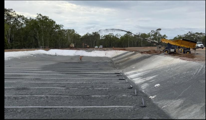
Lining of bio-retention ponds
