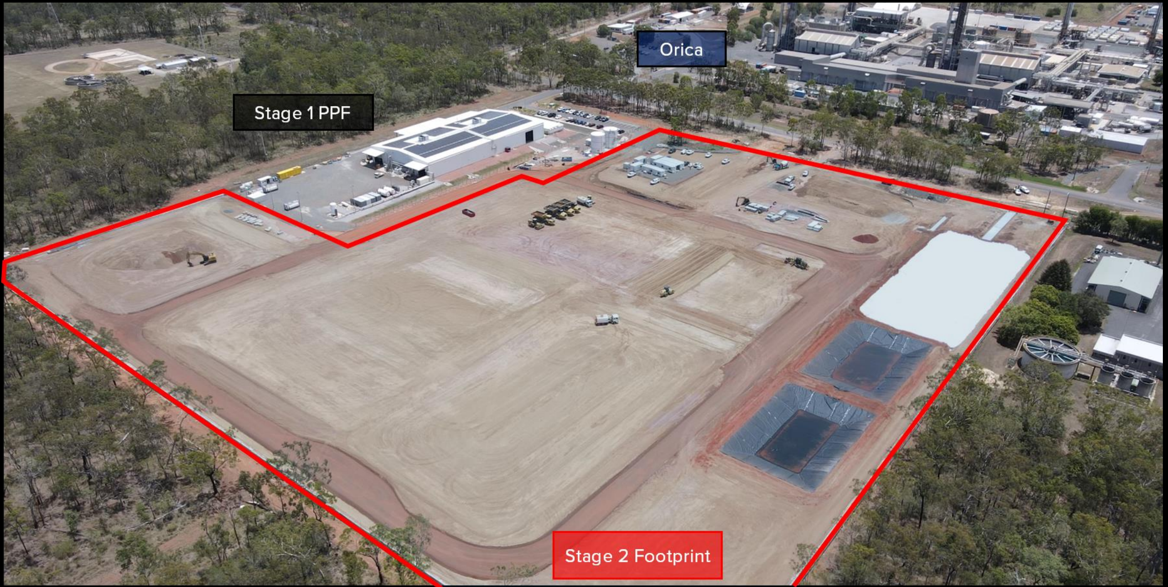
Stage 2 Bulk Earthworks – December 2024
