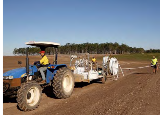
Laying infield irrigation pipe at Dowlings, Maryborough, Queensland, May 2023.
