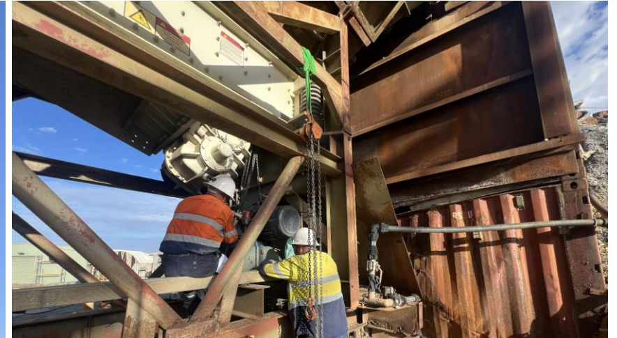
Primary crusher - pan feeder motor replacement underway
