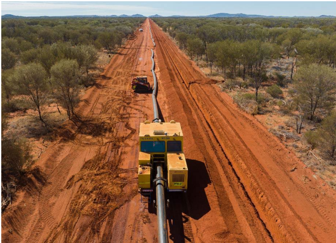
Installation of the arterial water pipeline between the Nolans borefield and the process plant site, June
