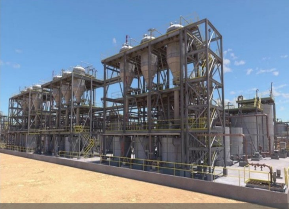
Rare earth extraction (candle filters)
