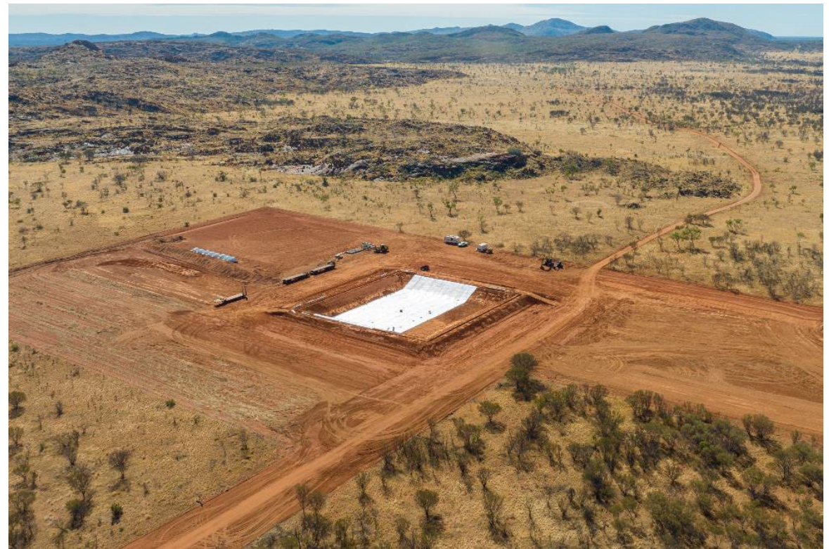
Aerial view of turkey nest dam installation, June
