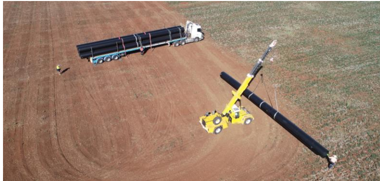
Delivery of 20 m long, 1 m diameter poly pipes for irrigation at Riverton (July 2022).
