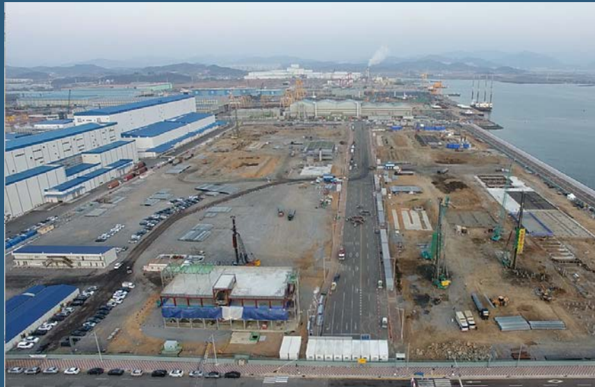
43,000tpa LHM facility under construction in Gwangyang, South Korea
