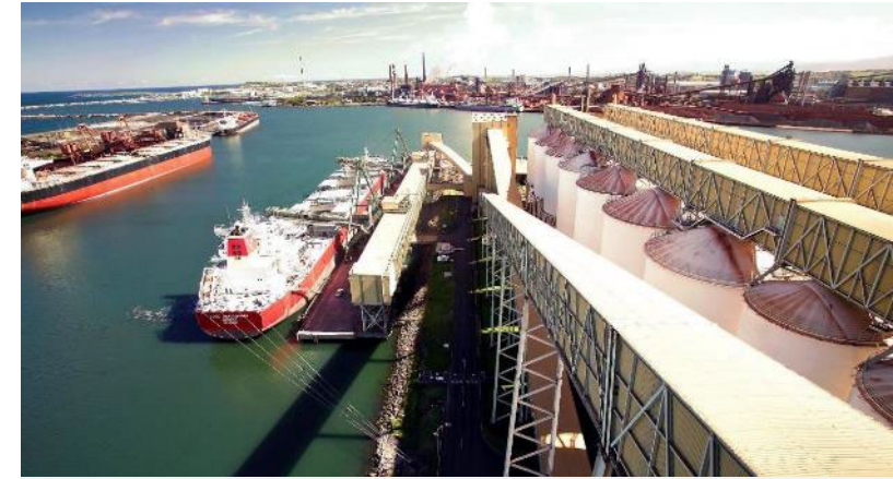
GrainCorp bulk port terminal, Port Kembla, NSW
