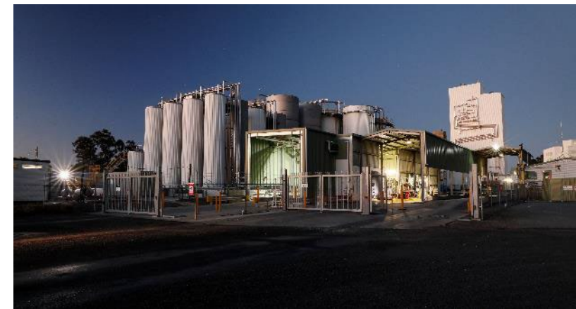
GrainCorp oilseed crush plant, Numurkah, VIC
