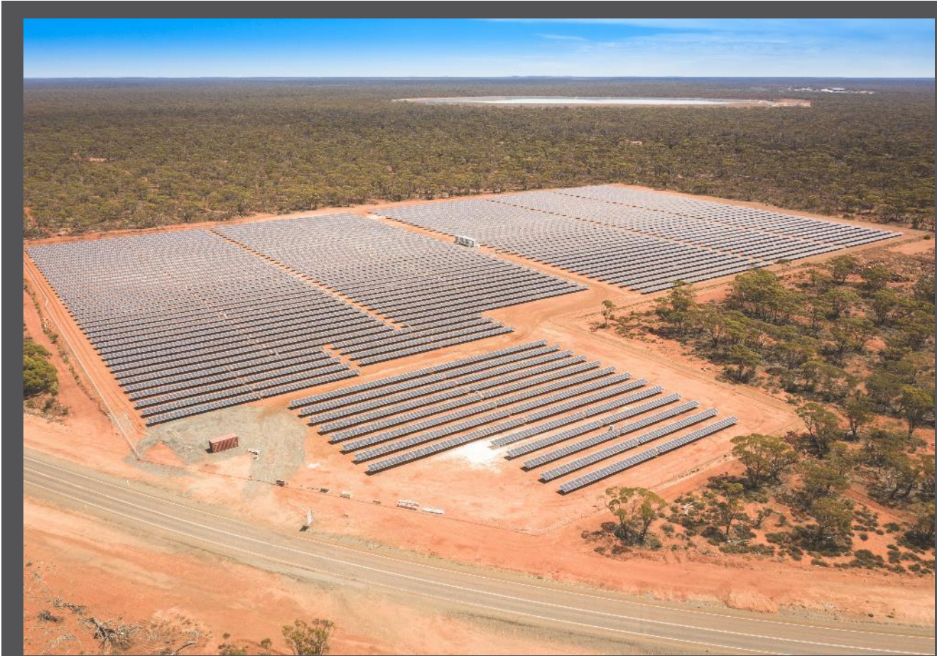
Zenith currently constructing 2MW solar energy and battery farm at KOTH (similar Zenith power installation shown in picture)
