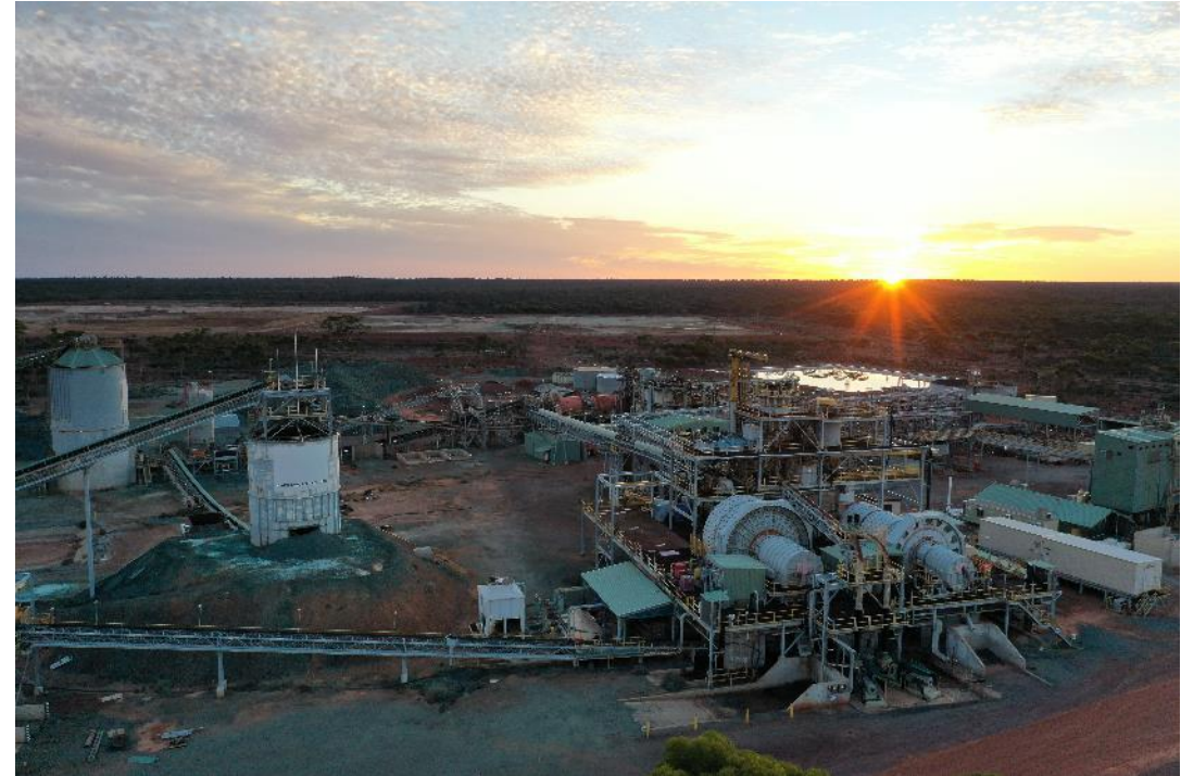
Black Swan 2.2Mtpa milling circuit Plans to refurbish and de-rate to 1.1Mtpa throughput
