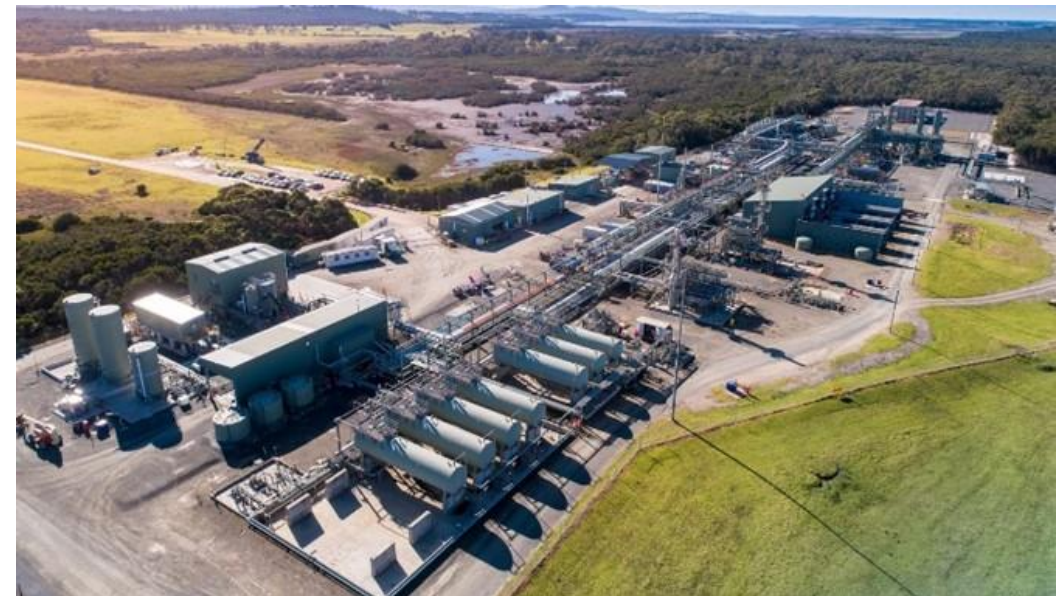
Orbost Gas Processing Plant, owned and operated by APA
