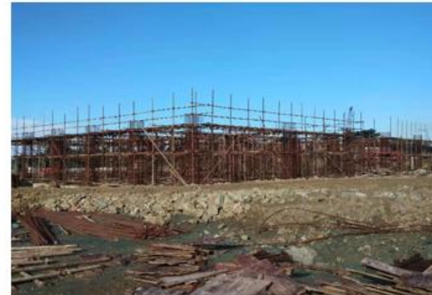
Column reinforcement for Electrostatic Precipitator
